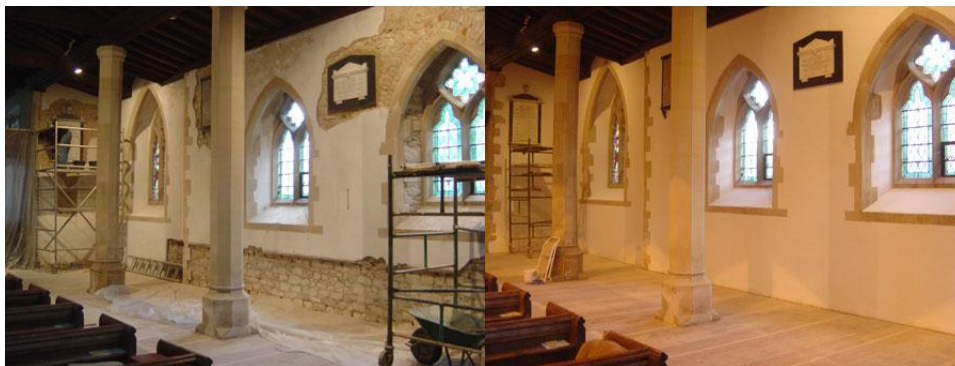
Lime plastering in a church
