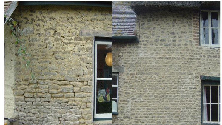
Lime pointing of Stonework
