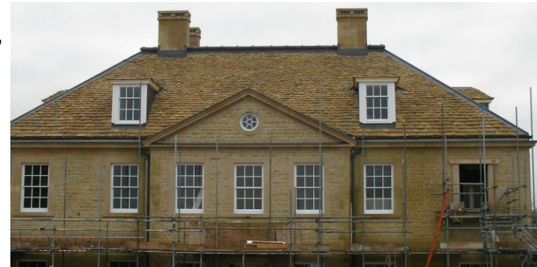
Roof using Cotswold random stone and a variety of lead works.
